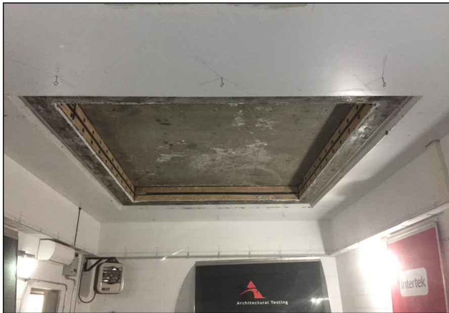
Receive Room View of Test Specimen Installation
